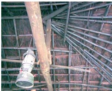
Fig. 28. Bamboo beams &thatched roof
