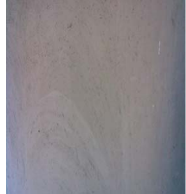
Fig. 21 .Floor cladding with Dung & Husk
